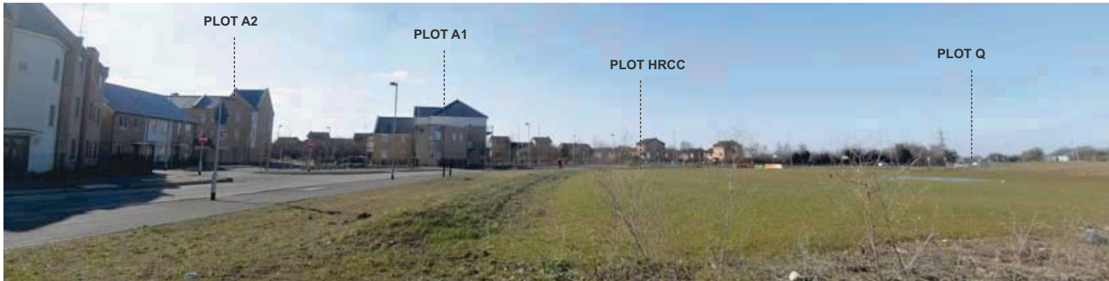
FIG 9 - PANORAMIC VIEW 9 (LOOKING SOUTH)
